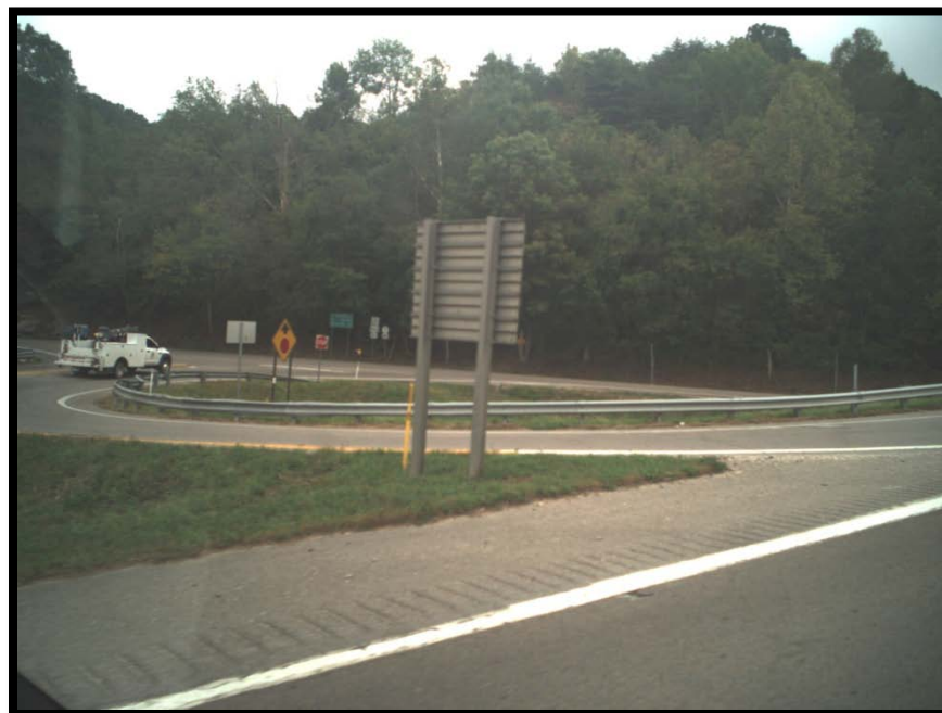
Figure 7: Cloverleaf Exit Ramp onto KY 7
