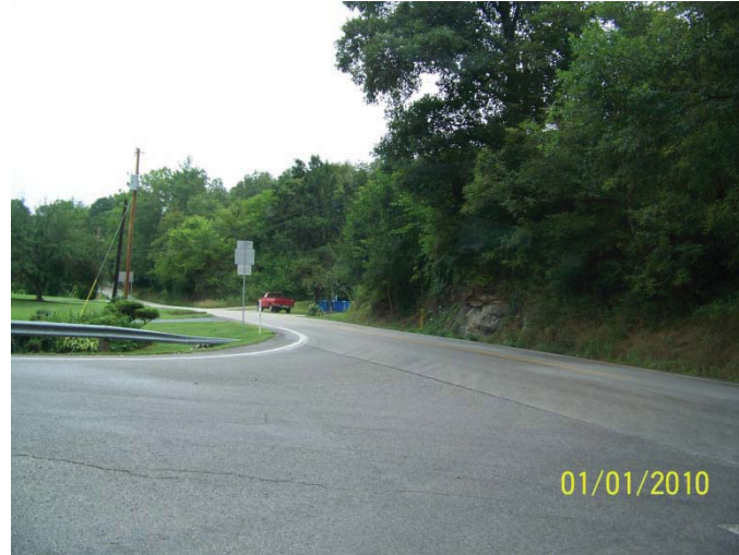
Looking NW from Exit Ramp on KY 7
