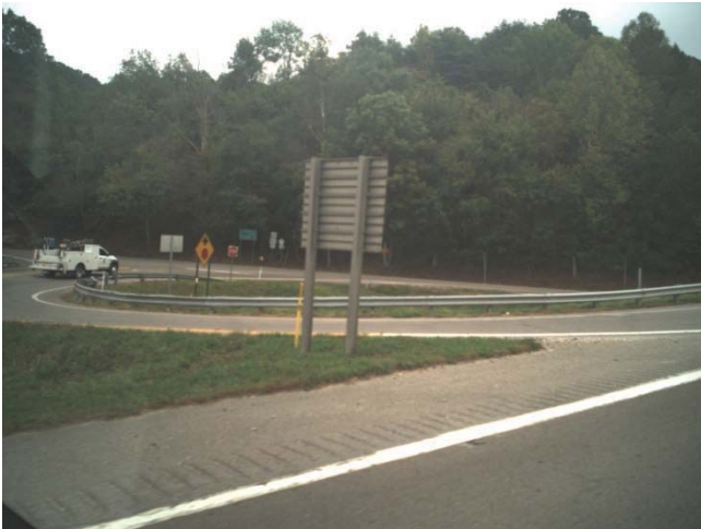
KY 9009 Westbound Exit Ramp
