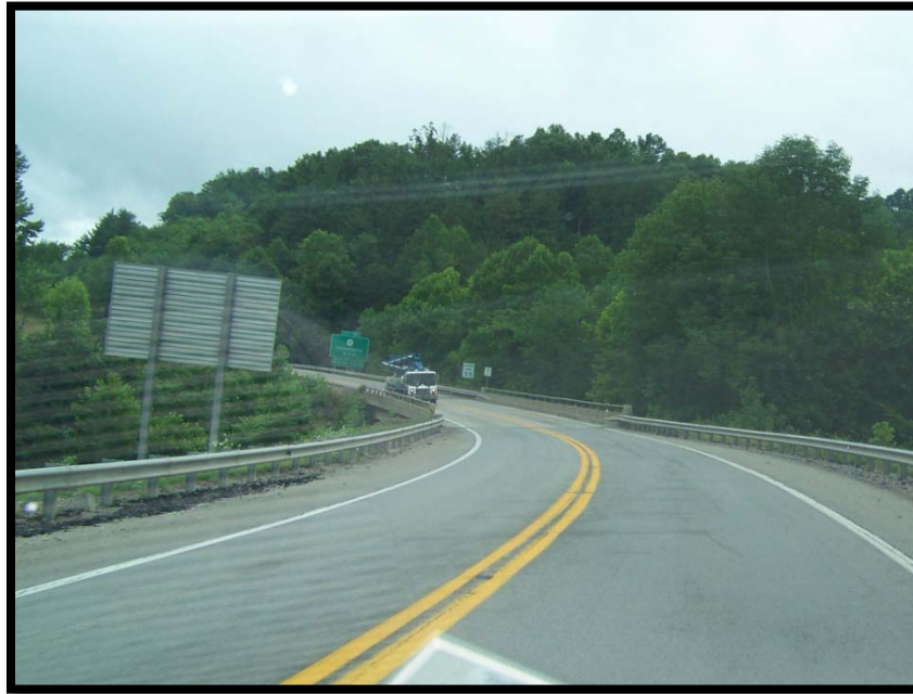
Figure 5: Bridge over Burning Fork
